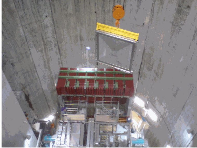
Figure 4.3: Installing the FGD. The crane slowly lowered the FGD into the basket.
